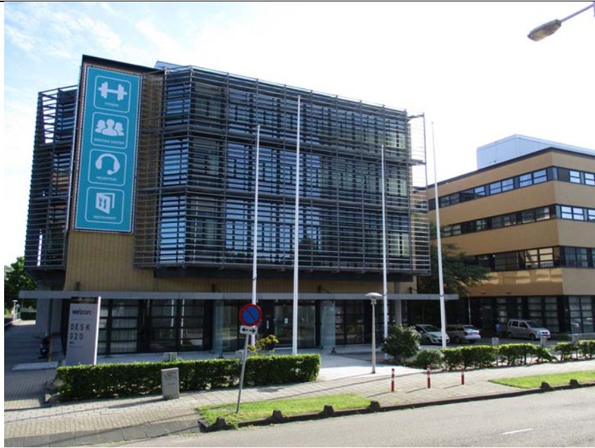
Photo 3. View towards the north, Verizon office building
