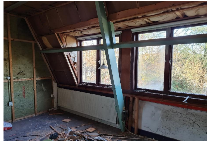
Verdieping met later aangebrachte dakkapel (1979)
